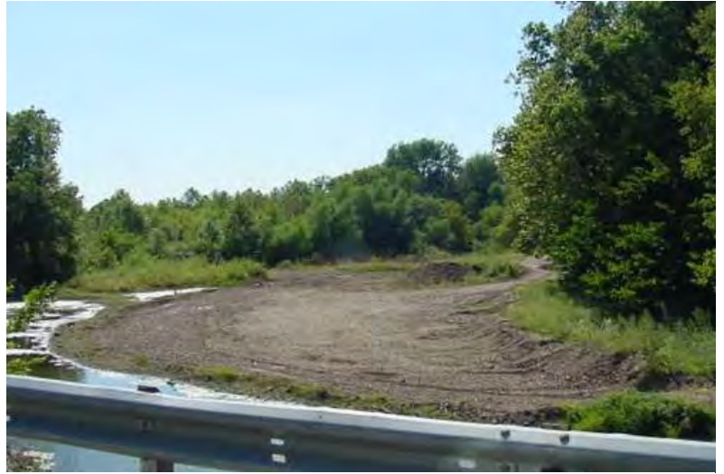
Gravel is best removed from loosely packed bars above the water. Leaving undisturbed buffers helps minimize impacts to stream stability, water quality, and aquatic health.
