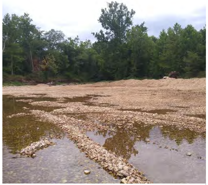
Improperly removing gravel from below the water decreases stream stability and destroys aquatic habitat.
